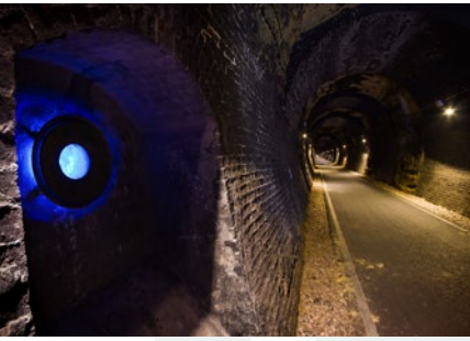
The tunnel could be transformed from a decaying relic into a socially useful asset, like Combe Down Tunnel in Bath.
