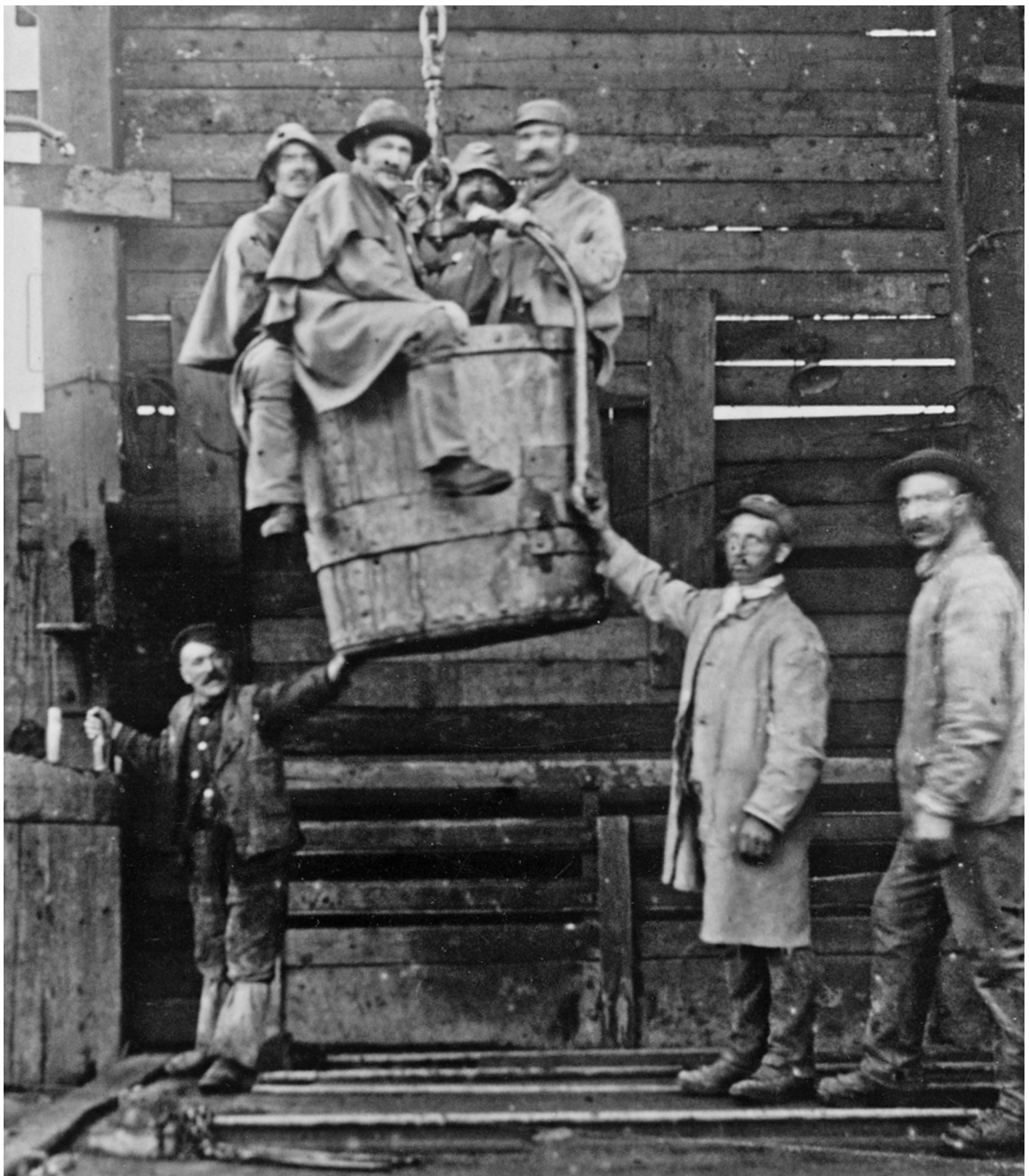
Navvies prepare to descend a shaft during the construction of Cowburn Tunnel near Chinley in 1894.
