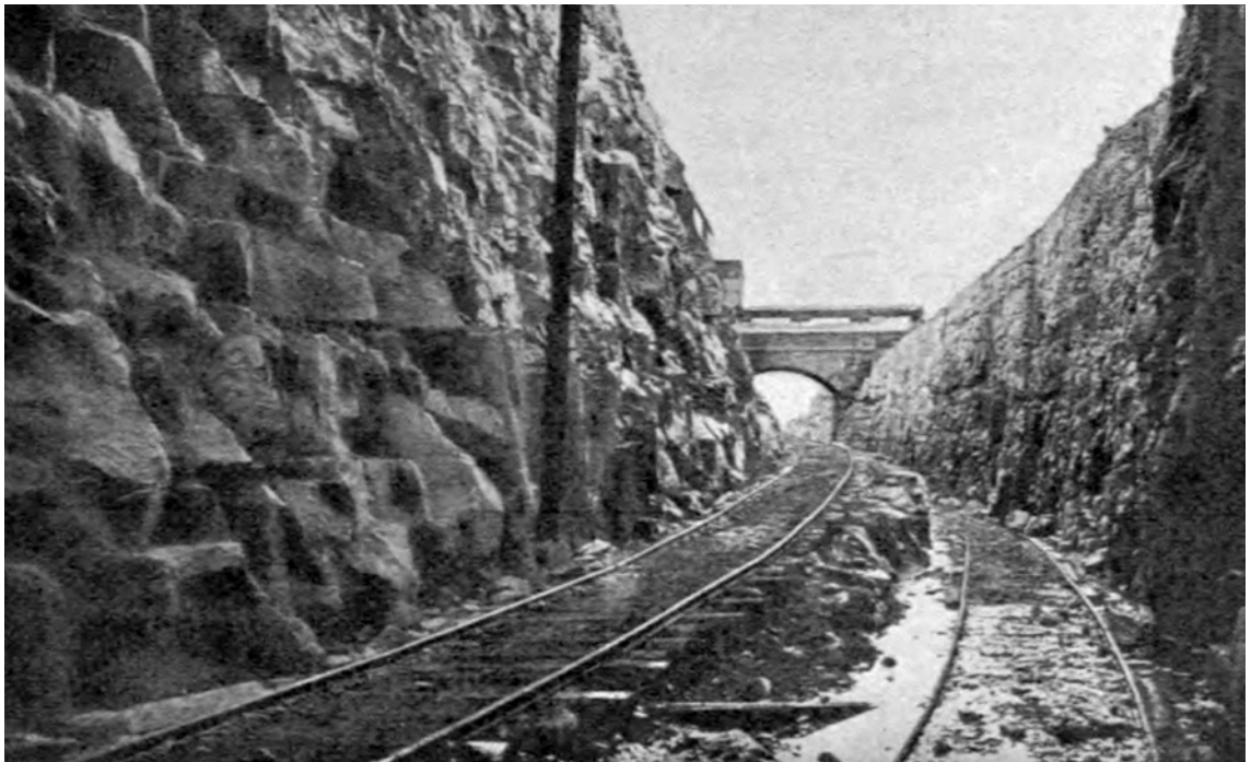
The view from the southern entrance of Queensbury Tunnel into the approaching cutting during its excavation.
